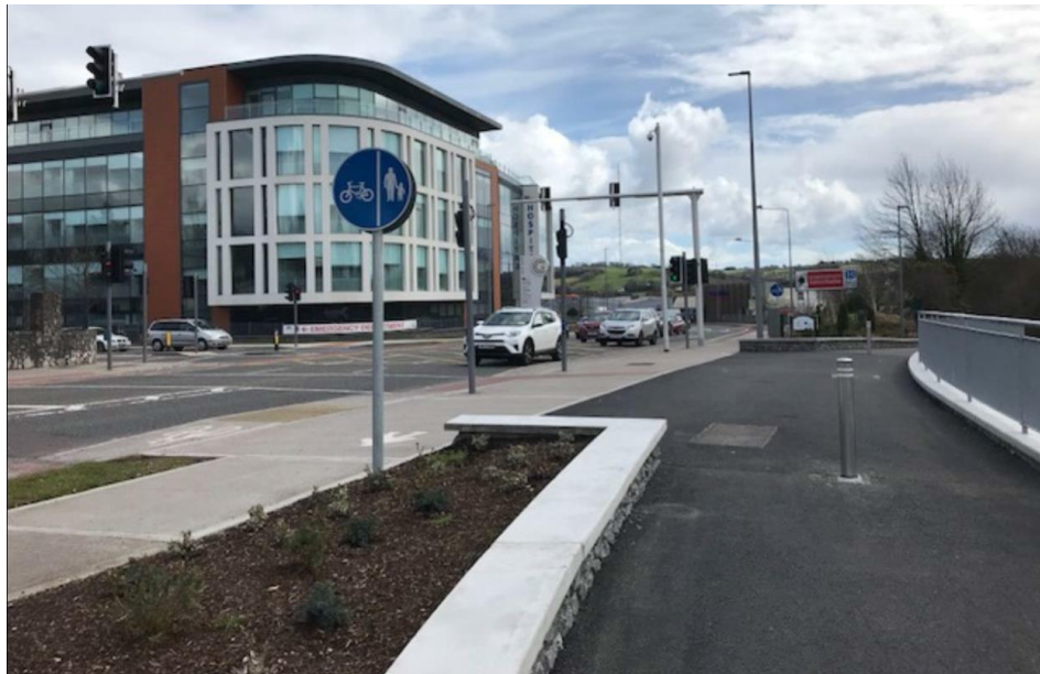
Figure 20 New Cycle Ramp access at junction of Mahon Link Road and St. Michael's Drive
