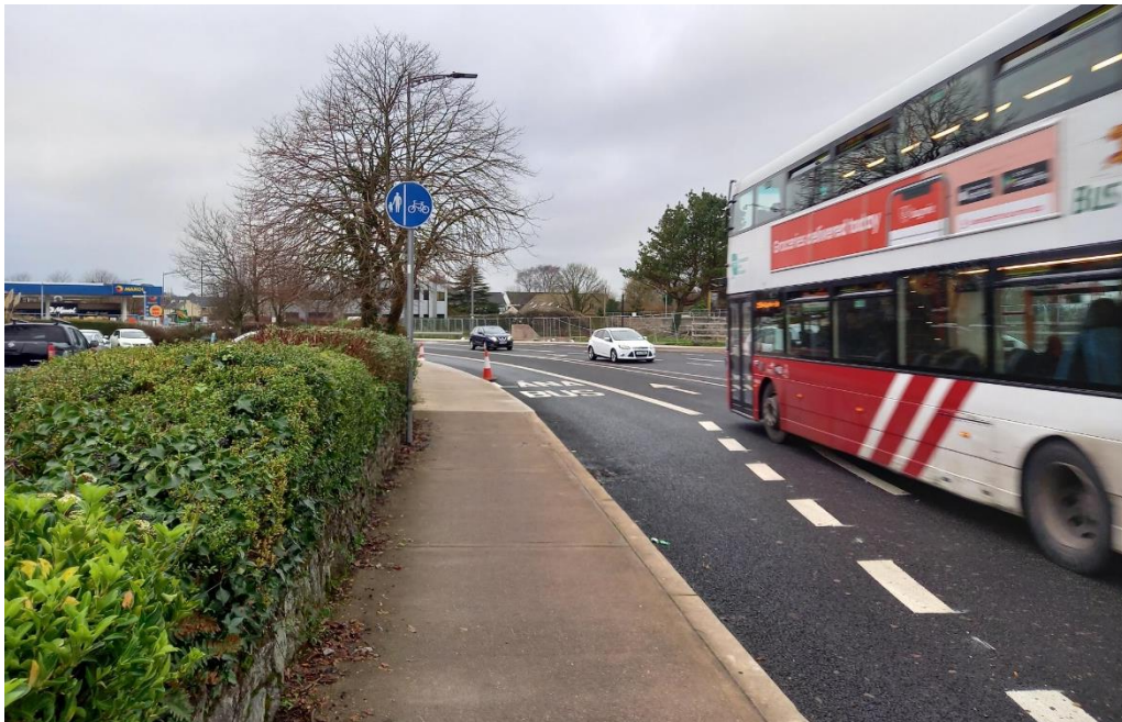
Figure 32 New bus lane on Skehard Road
