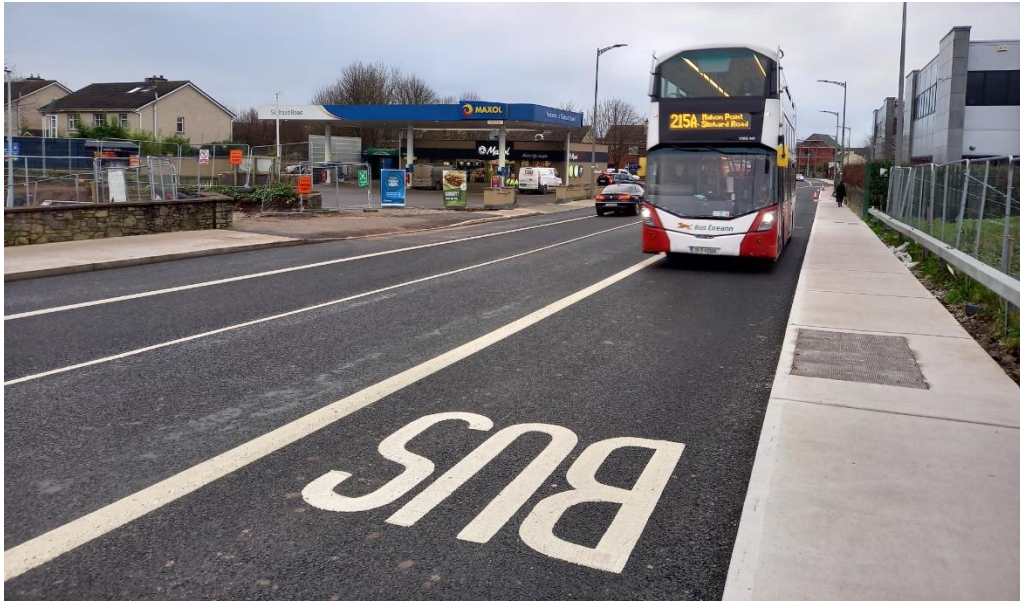
Figure 31 New bus lane on Skehard Road
