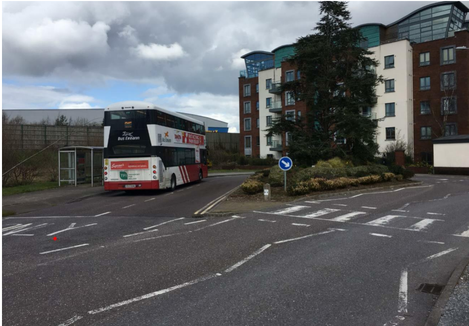
Figure 23 Existing Bus Terminus and Turnaround Area at The Sanctuary, Jacob's Island
