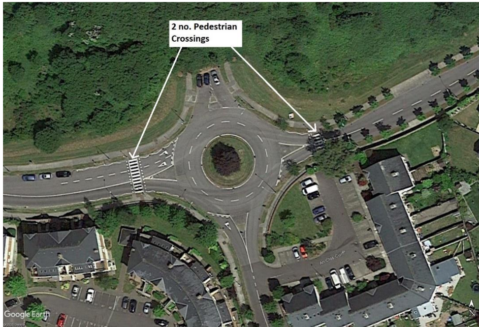
Figure 11 Roundabout Junction at Jacob’s Island
